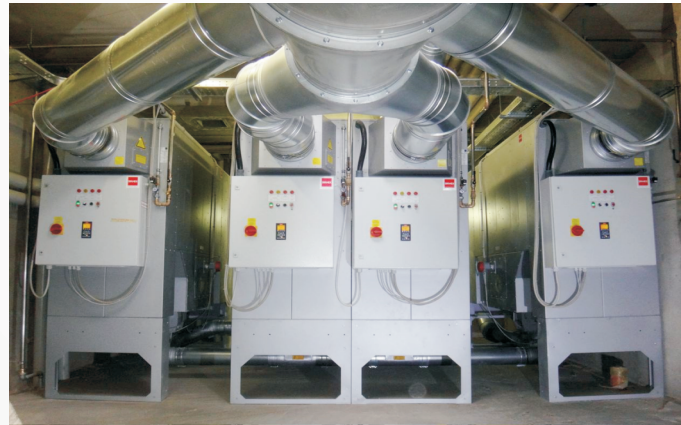
Image 1: Air quantity capacity 40,000 m 3 /h
