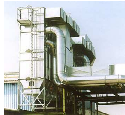
line filter with reverse-air cleaning
